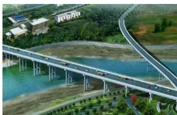
(a) 水上桥梁1 (a) Water bridge 1
