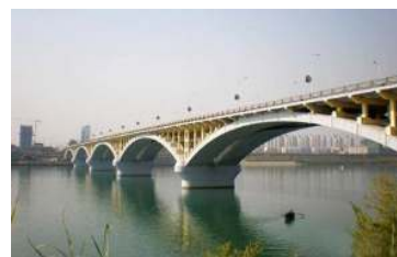
(c) 水上桥梁3 (c) Water bridge 3
