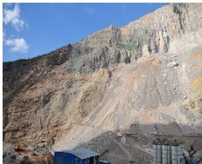
(a) 监测现场 (a) Monitoring site
